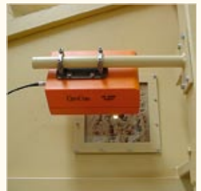
Side wall of dosing bin
