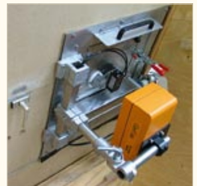
FMV in drop chute underneath dryer cyclone
