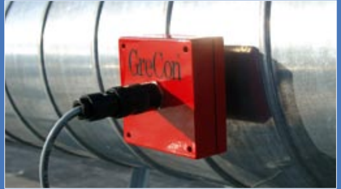
Mounted spark detector
